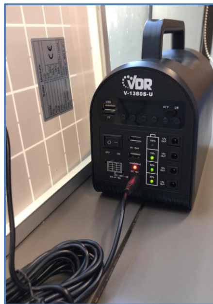
Figure 2. Solar Panel and Battery Tests
